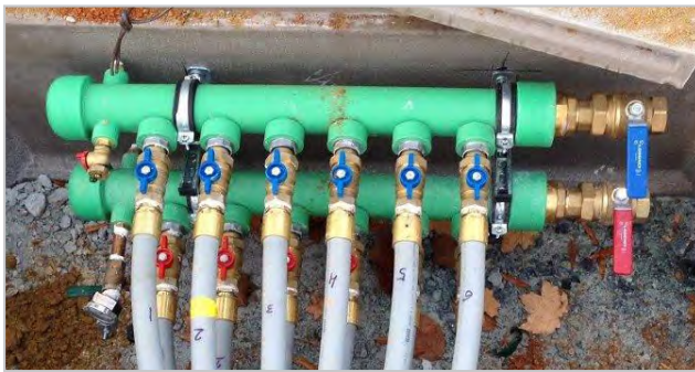
M-8400 GeoGreen™ mounted ground vault.
