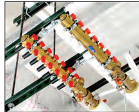
All Legend brass manifolds can be mounted at any orientation
